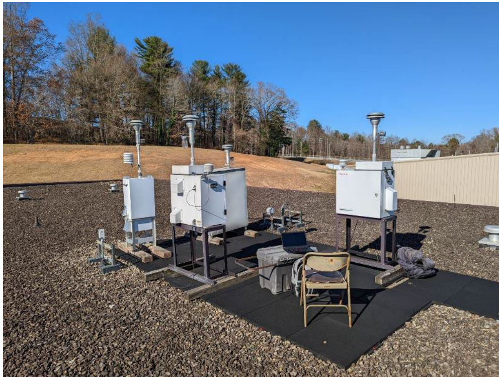
Previous roof top site
