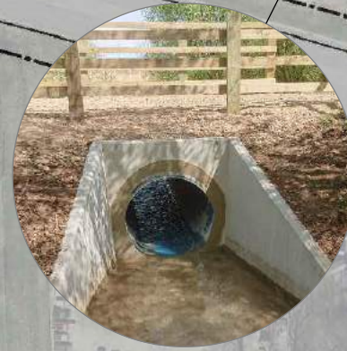
PEDESTRIAN CULVERT BRIDGE
